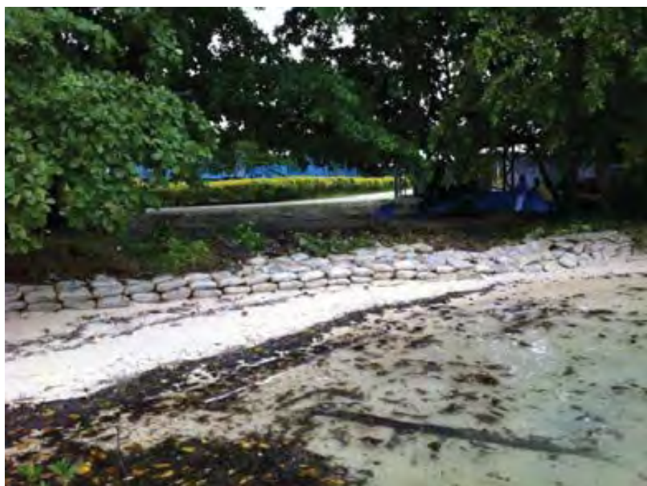
Figure 2-7 Sand bag wall preventing erosion on eastern side of Taro Island. Taro hospital is blue building in the background. Tide condition estimated to be mid-tide
