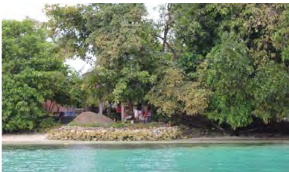
Figure 6-36 Coral rock breakwaters protecting individual properties on the north-east corner of Taro Island. View from west.
