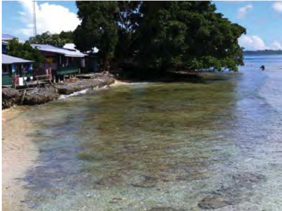
Figure 2-8 Coral gabions protecting and underpinning houses on the south-east corner of the island, adjacent E-S beach lodge. View to north. Low-mid-tide conditions
