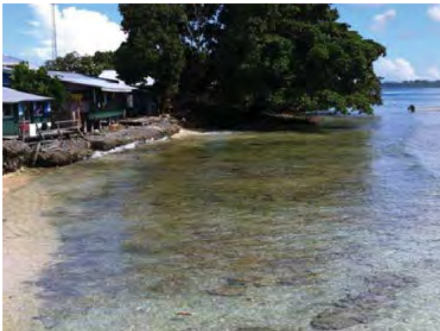
Figure 6-35 Coral gabions protecting and underpinning houses on the south-east corner of the island, adjacent E-S beach lodge. View to north. Low-mid-tide conditions.
