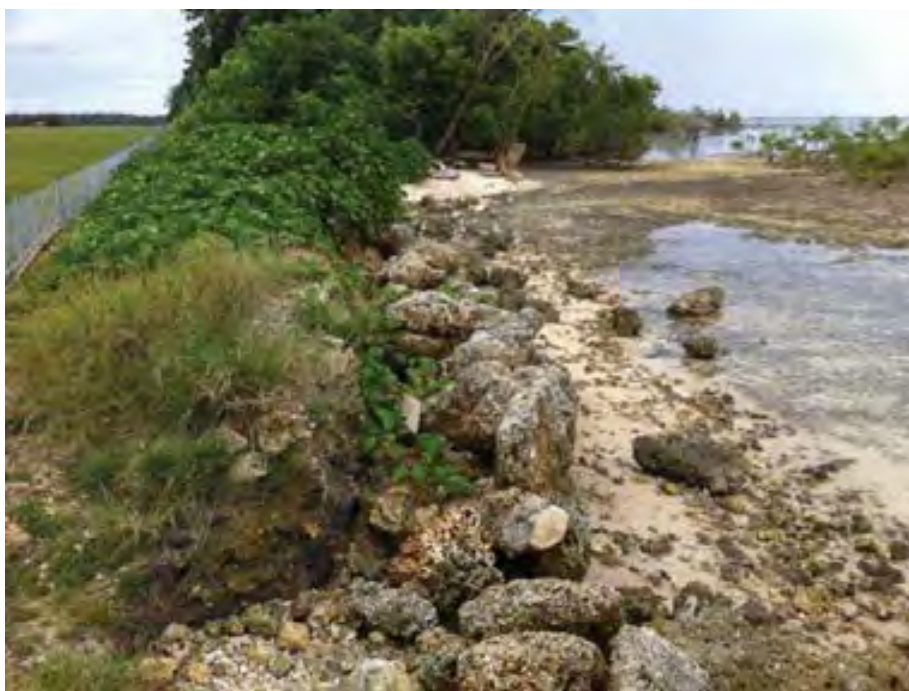
Figure 6-38 Coral boulders protecting runway on western (ocean) side of the island, northern end of the island. View to south
