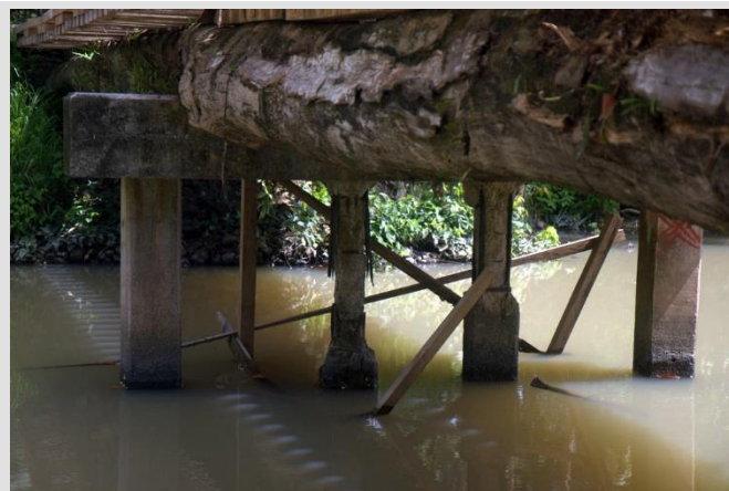
Plate 14: Detail of the underside of the Bora Bridge. Even though the bridge deck has been refurbished, the foundations have not been upgraded, and show signs of significant
