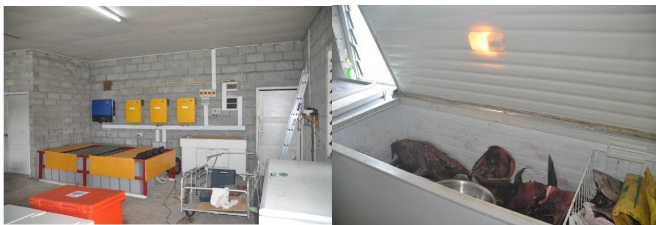
Figure 14: Ice plant inverters and batteries and energy use freezers – Teraina island Council
