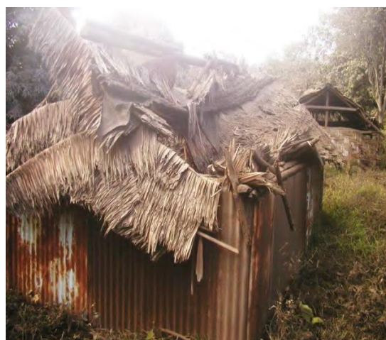
Fig. 16: House damaged by ash fall in Luli
