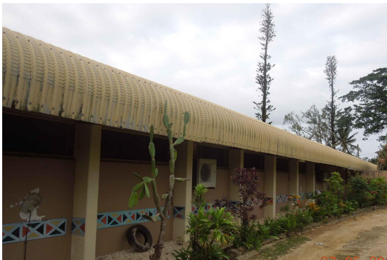
Fig. 14: An example of « building back better ». After Cyclone Uma in 1987, the Vanuatu Curriculum Development Unit was constructed with a rounded roof. The building suffered hardly any damage from Cyclone Pam. Photograph taken on 27th May 2015, two months after the cyclone.
