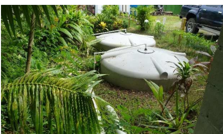
WAY FOR FUTURE: Biogas sanitation system creating energy from primary digester tanks to storage bags to BBQ oven. Located at the Samoa Cultural Village.
