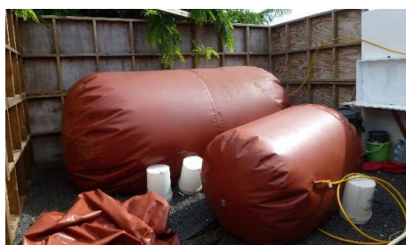
WAY FOR FUTURE: Biogas sanitation system creating energy from primary digester tanks to storage bags to BBQ oven. Located at the Samoa Cultural Village.
