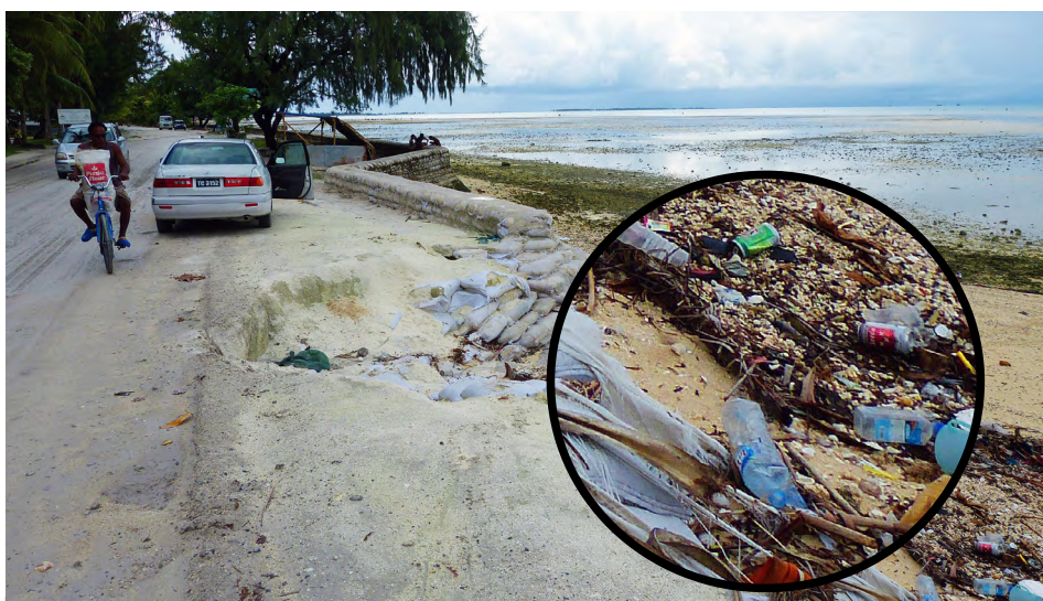
NOT PRETTY: Coastal erosion adjacent to a hard seawall in Tarawa, Kiribati.
