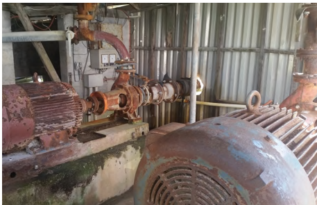
IN NEED OF REPAIR: Pumping mechanism in reverse osmosis desalination plant needs refurbishment. Photo by C-CAP
