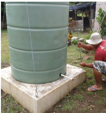
STABILITY IN SOPU, TONGA: A villager checks the cables that stabilize a new water harvesting tank in Sopo.
