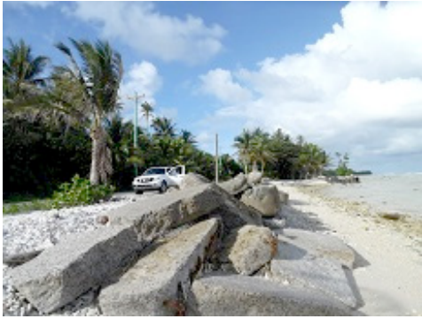
FIGURE 2. ROAD EXPOSED TO OVER-WASH
