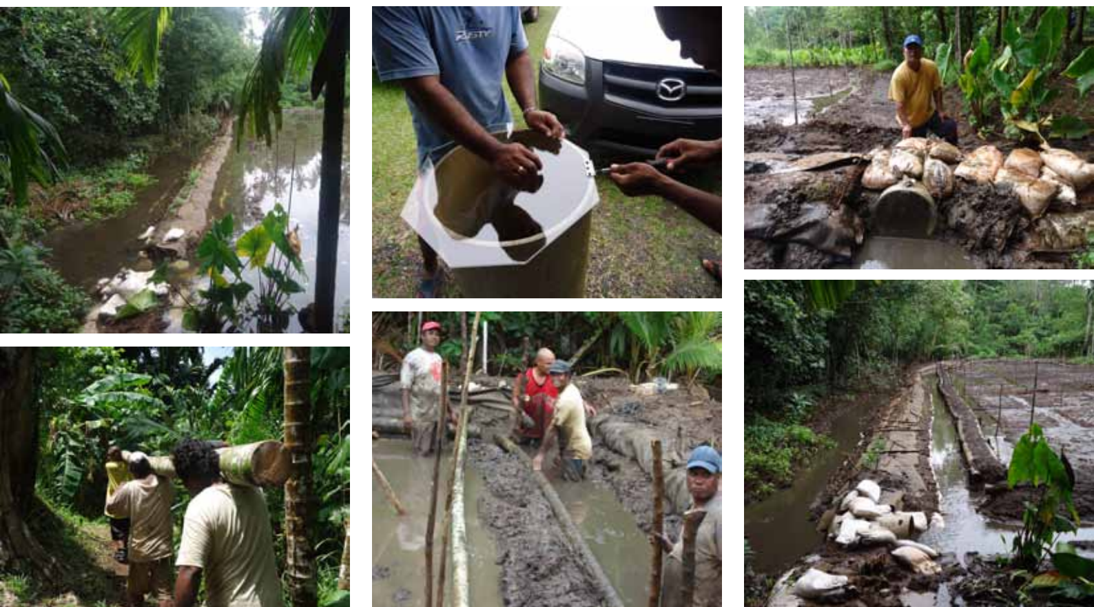
An adaptation project in Palau: Construction of a dike system in a taro patch to reduce the impacts of sea level rise, coastal erosion, flooding, and salt water intrusion © PCC.
