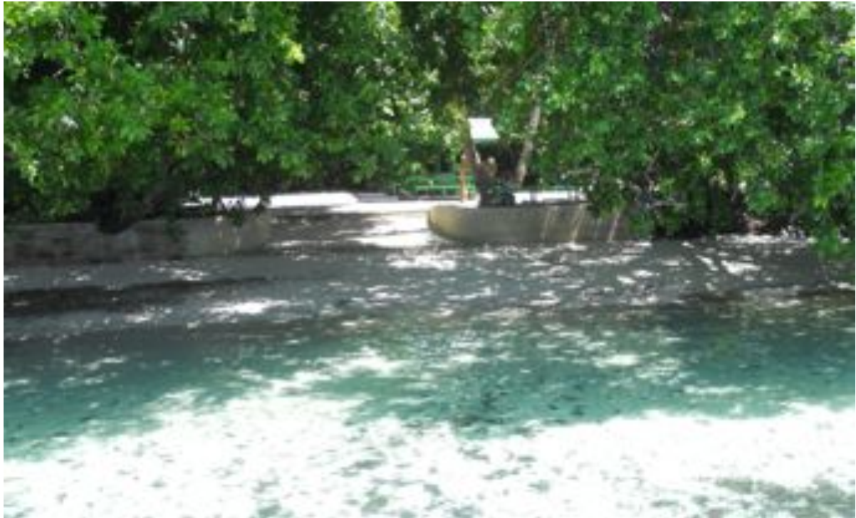
Site 4. Located near Ngermeaus Beach with an easterly aspect this north / south running beach has been subject to hard vertical seawall construction. There was low sand accumulation in front of the wall and exposed beach rock can be seen to the left. Vertical walls tend to reflect wave energy and frequently push sand away rather than allowing it to deposit on the shore.
