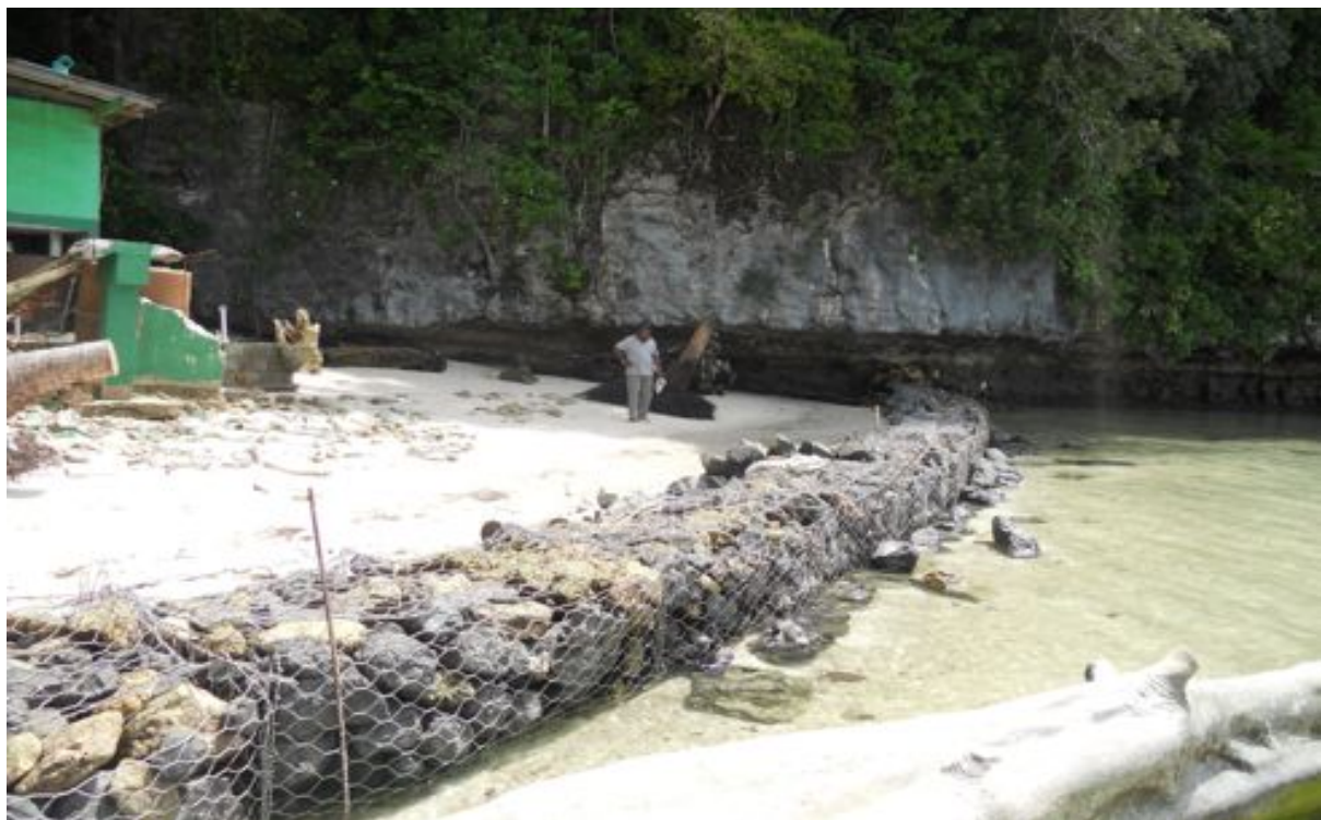
Protective gabion basket wall and remains of one of two compost toilet facilities to the left. The wall approximates the former berm position.
