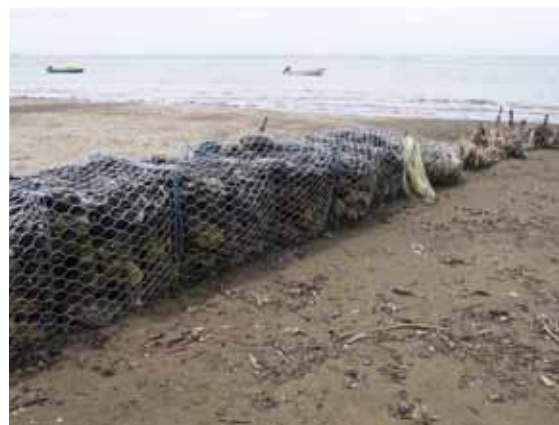
Plate 5. A local attempt to build a groyne to slow down rapid coastal erosion. This groyne made from gabion wire and rocks fell apart in less than two years. The other side of the groyne experienced rapid erosion after it was built.
