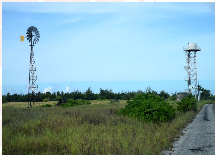
Wind energy technology to draw water from the ground
