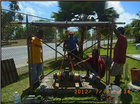
Bulk Meter installed at the RMI Airport Reservoir. Photo: MWSC
