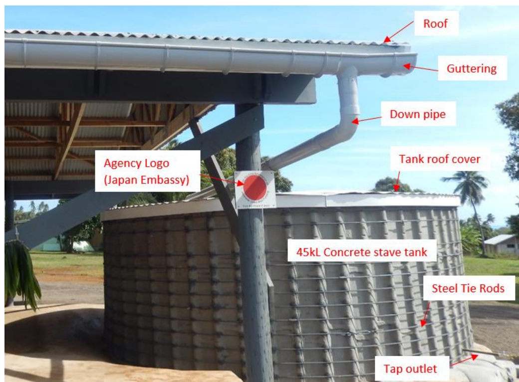
Figure 10. Typical Pa Enua Community 45kL Concrete Water Tank
