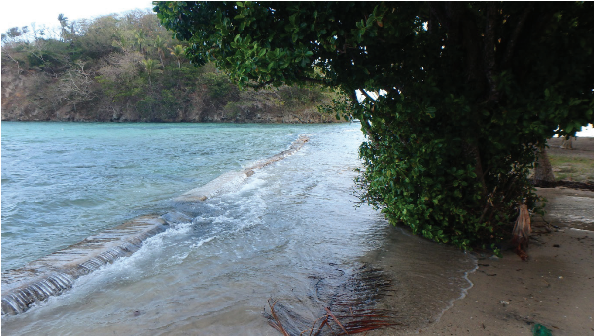
Photo B4. Extent of damage to seawall at low tide (Photo: James Jolliffe)
