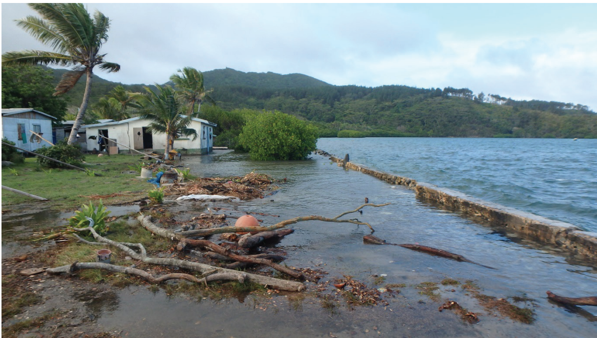
Photo B2. Breached seawall at high tide (Photo: James Jolliffe)
