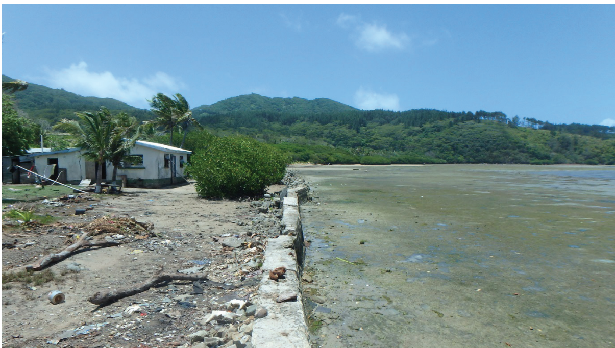
Photo B4. Extent of damage to seawall at low tide (Photo: James Jolliffe)
