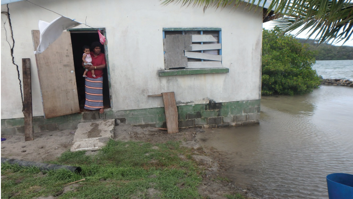
Photo B1. Front Line household at high tide. The householder believes that the thick crack to the left is caused by the house sinking due to inundation. (Photo: James Jolliffe)
