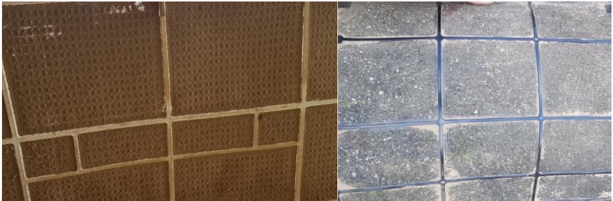
Figure 4-11: Examples of air filters from Tafunsak air conditioners before (left) and after (right) cleaning.
