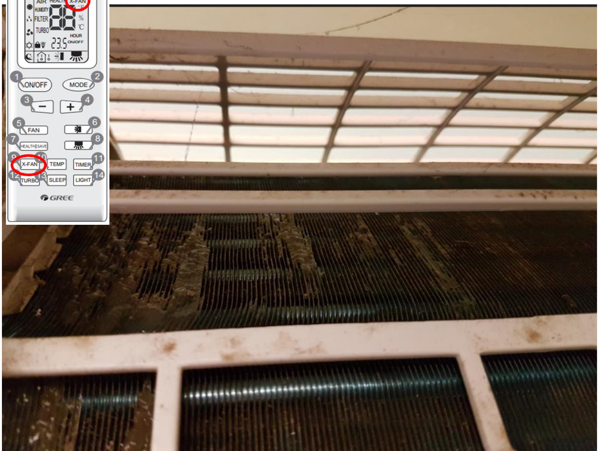
Figure 4-12: Sludge accumulated on evaporator coil of admin office air conditioner. selected in cooling or dry mode operation. This setting keeps the evaporator fan running for 10 minutes
