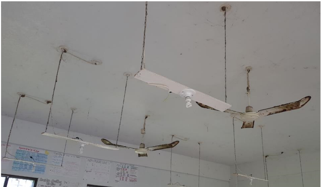
Figure-7-1: Typical CFL retrofit in KHS classrooms. A proper light fixture with reflector and/or diffuser would direct light output downwards, that is otherwise scattered to the walls and ceiling. Note also the condition of ceiling fans.
