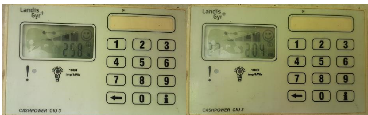
Figure-6-2: Cashpower keypad at Home Arts meter. Left picture shows present load (258W), accessed by entering 'i, 001' on the keypad. Right picture shows month-to-date energy consumption (204kWh) and days counted (27), access by entering 'i, 008'.
