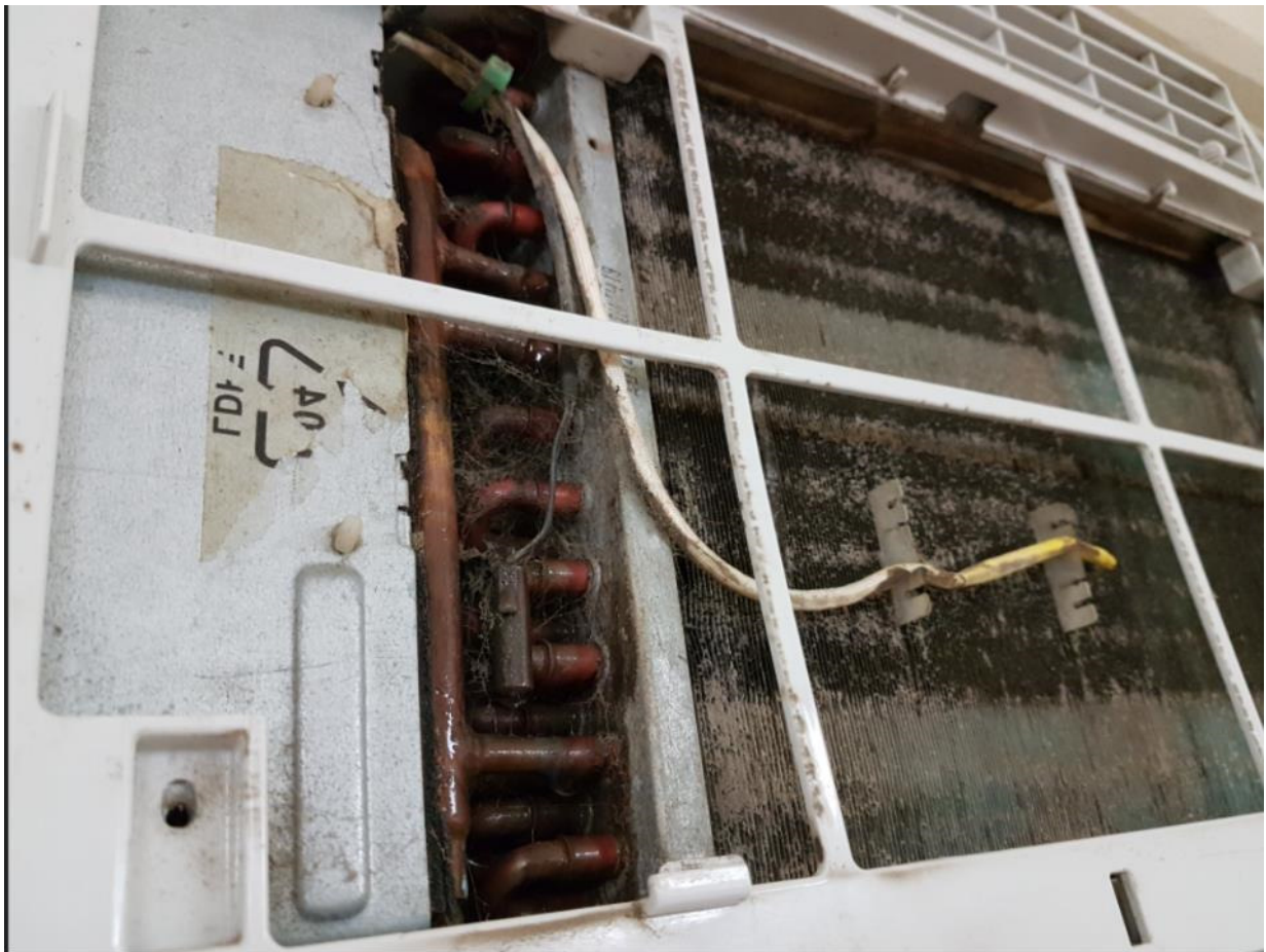
Figure 4-17: Dust build up directly on evaporator fins. Disassembly and cleaning by a qualified technician may be required.
