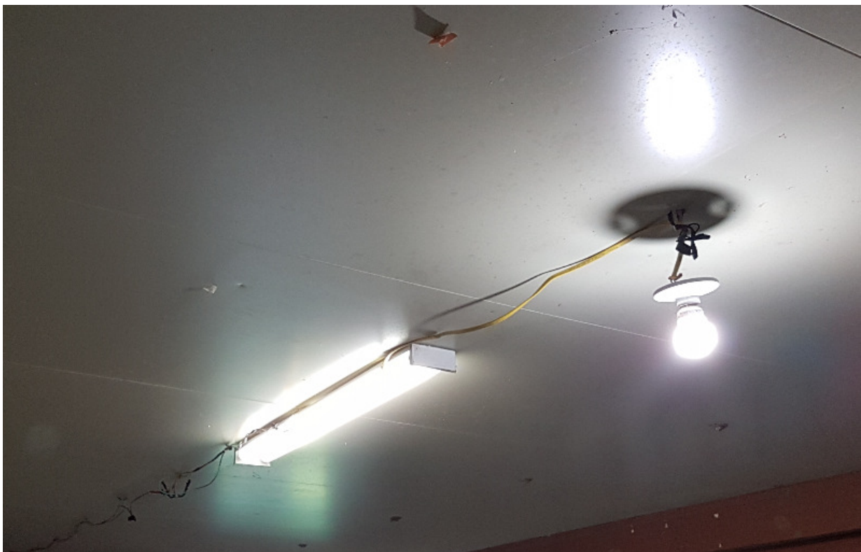
Figure 4-6: Example of lights and wiring in resource room (RNR). Illumination is inconsistent and utilisation factor is poor. Wiring presents a real safety and fire hazard which should be addressed.
