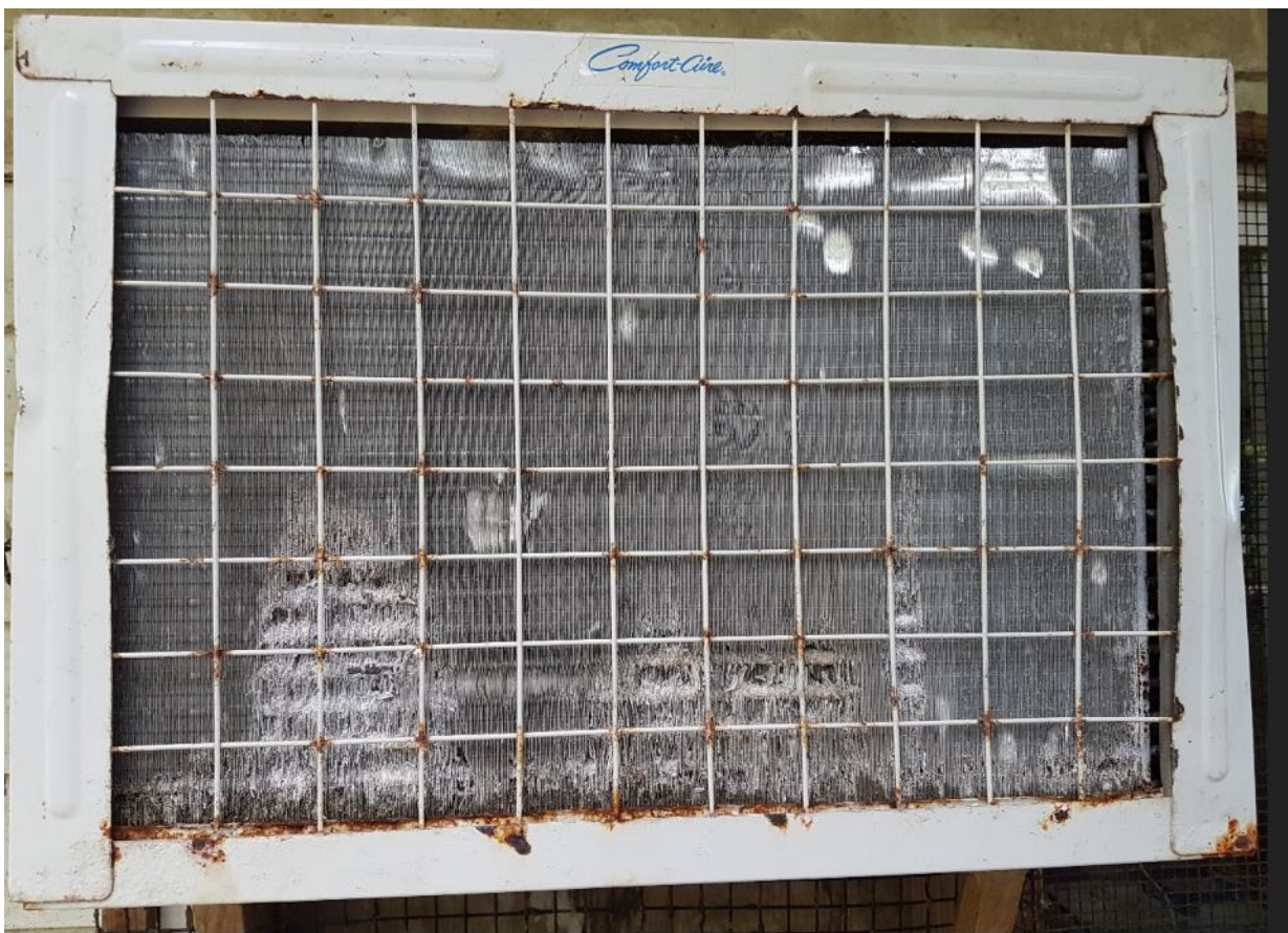
Figure 4-5: Condenser fins on RNR air conditioner (outdoor side).
