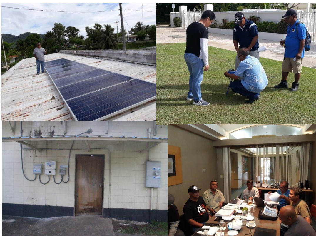
Photos: Left top and bottom: Kosrae 3.25 kW installation with inverter and net meter at KUA administration building Right top and bottom - Participants at the Solar PV grid connected training in Guam
