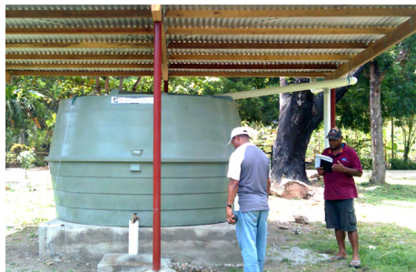
CATCHING RAIN: Inspecting the new rainwater catchment structure in Papua New Guinea.
