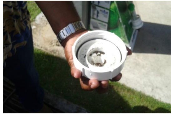
Mr. Ray Tamow showing the dirt particles captured by the first-flush device
