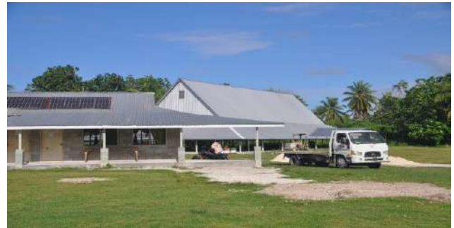
Figure 10. Tabuaeran Island council office and maneaba installation – 10 kW solar system
