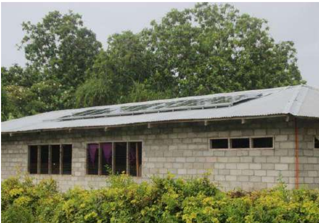
Figure 9. 5kw Solar panels roof mounted on both sides
