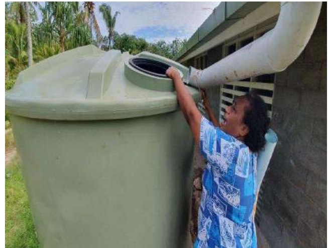
Figure 12. Water tanks inspected at the Teraina Primary school
