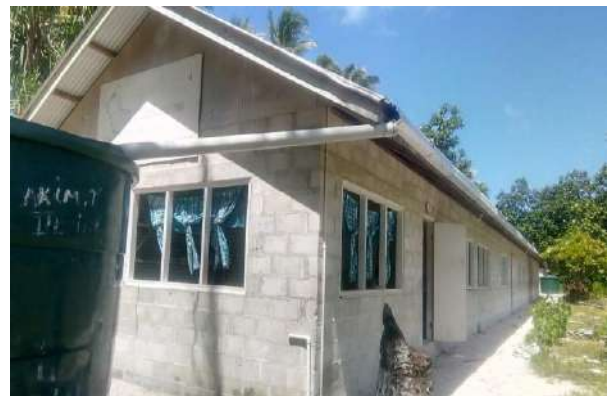
Figure 13. Installed water cutters and pipes at Tabuaeran JSS
