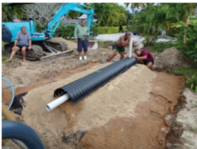
Drain layer professionals installing the land application bed for a wastewater system in the Lagoon Protection Zone of Muri.
