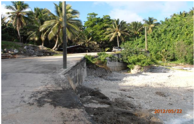
Figure 2 Sea wall at Avatele Ramp
