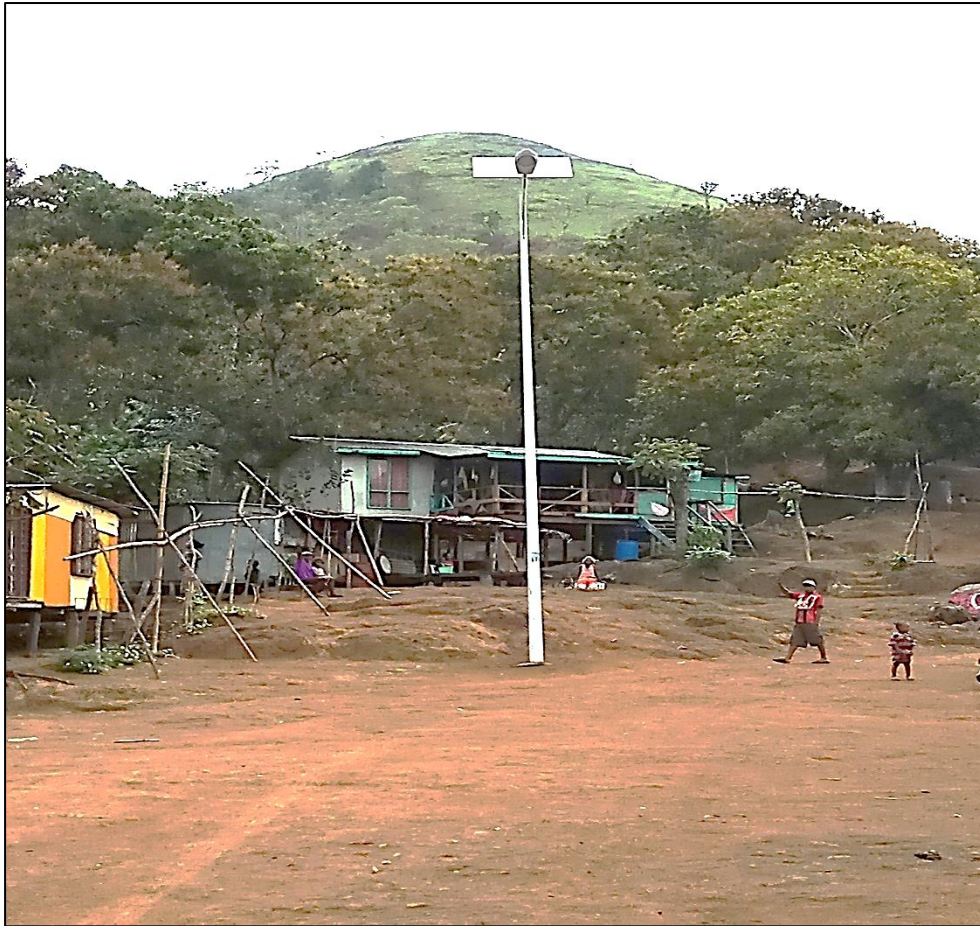
Figure 21 Solar street light in Imuagoro
