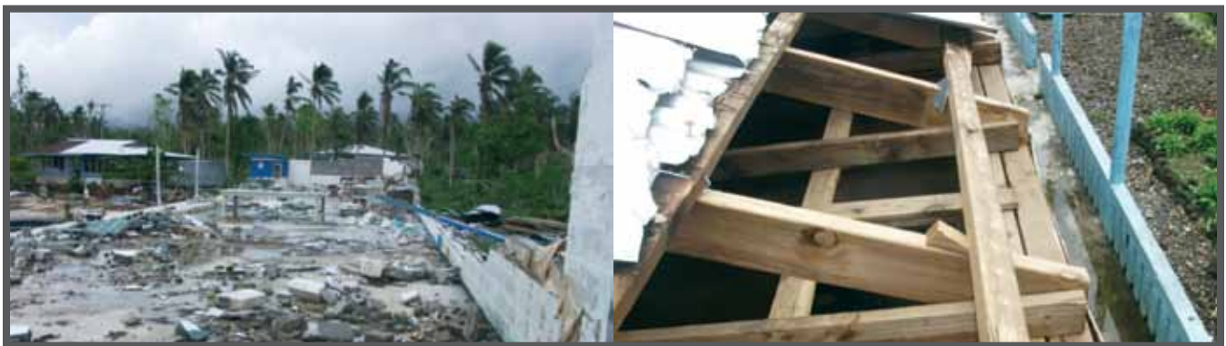
Photos Left: Salamumu Primary School, total rebuild required from foundations up. Right: Faleseela Primary School, Strengthening required for roof structure tie downs. Courtesy of GoS/PDPA Assessment team.
