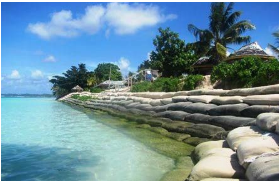
SAMOA: Completed coastal revetment in Manase.
