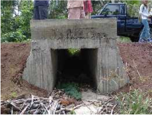
Figure 26. Box culvert from concrete and pipe culvert from corrugated metal sheeting
