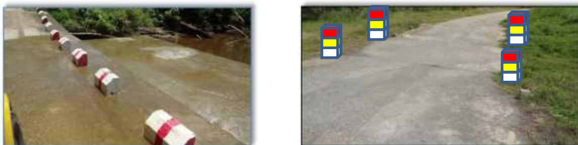
Figure 66 – Concrete warning blocks on drift
