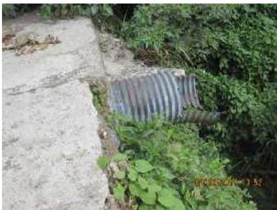
Figure 32. Cross drainage poorly maintained
