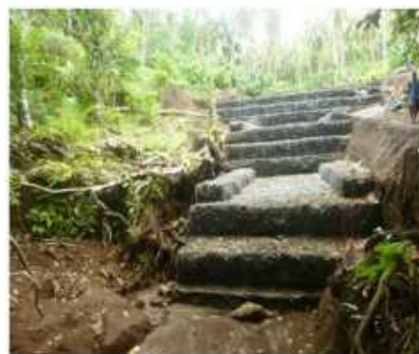
Figure 68 – Scouring under road and gabions for energy dissipation
