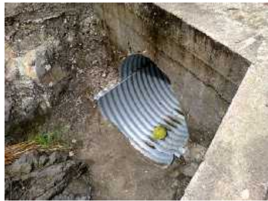
Figure 26. Box culvert from concrete and pipe culvert from corrugated metal sheeting
