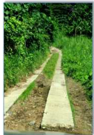
Figure 53. Concrete strips
