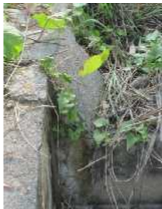
Figure 32. Cross drainage poorly maintained
