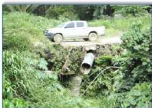
Figure 67 – Flumed drift (culvert under drift) requiring maintenance
