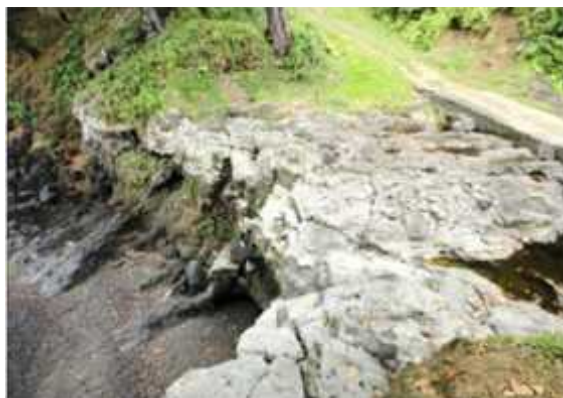
Figure 68 – Scouring under road and gabions for energy dissipation
