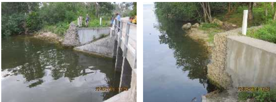
Figure 33. Gaions used in water crossings
