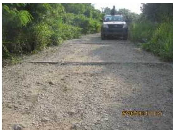
Figure 37. Horizontal scour checks
