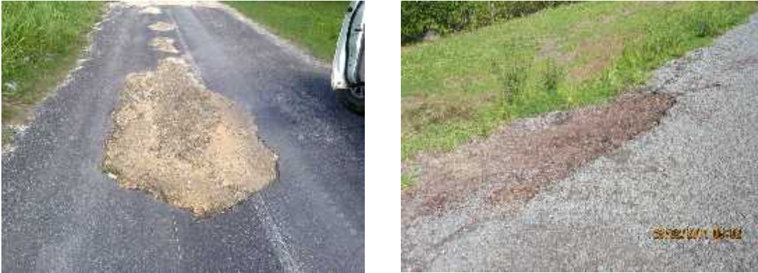
Figure 16. Pavements and Shoulders Breaking-up
