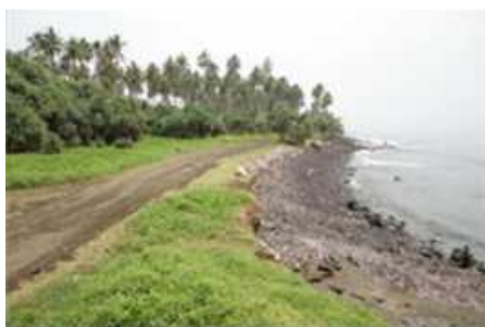
Figure 49. Evidence of Coastal Erosion
