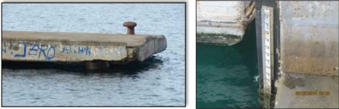
Figure 51. Wharf with low freeboard at high tide. Tide Gauge
