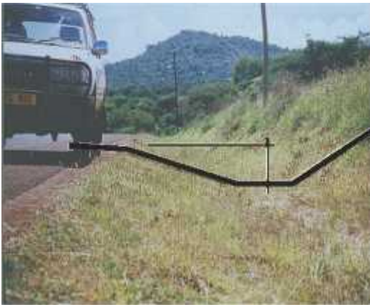
Figure 20. Minimum crown height
